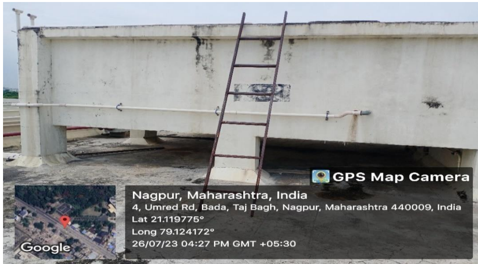
Overhead Water Tank
